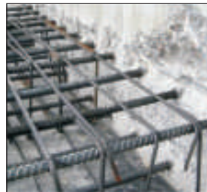
Beam to column connection
