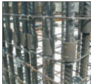
Wall to slab connection
